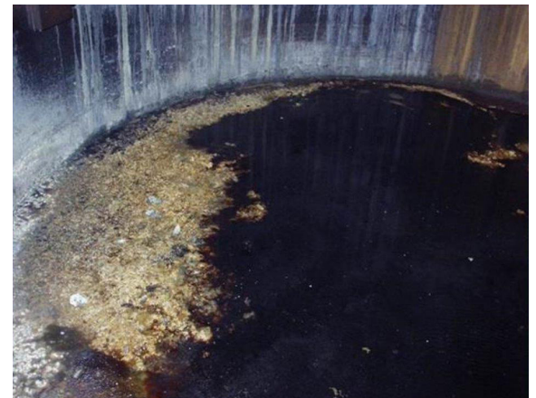
Stack Corrosion
