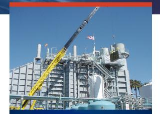
VOGT POWER SOLUTION Vogt performed Turnkey construction to decommission harps, add harps, modify harps to new service, and add catalyst.
